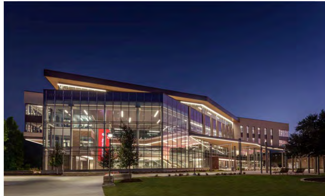
Wayne Roberts '85 Building
